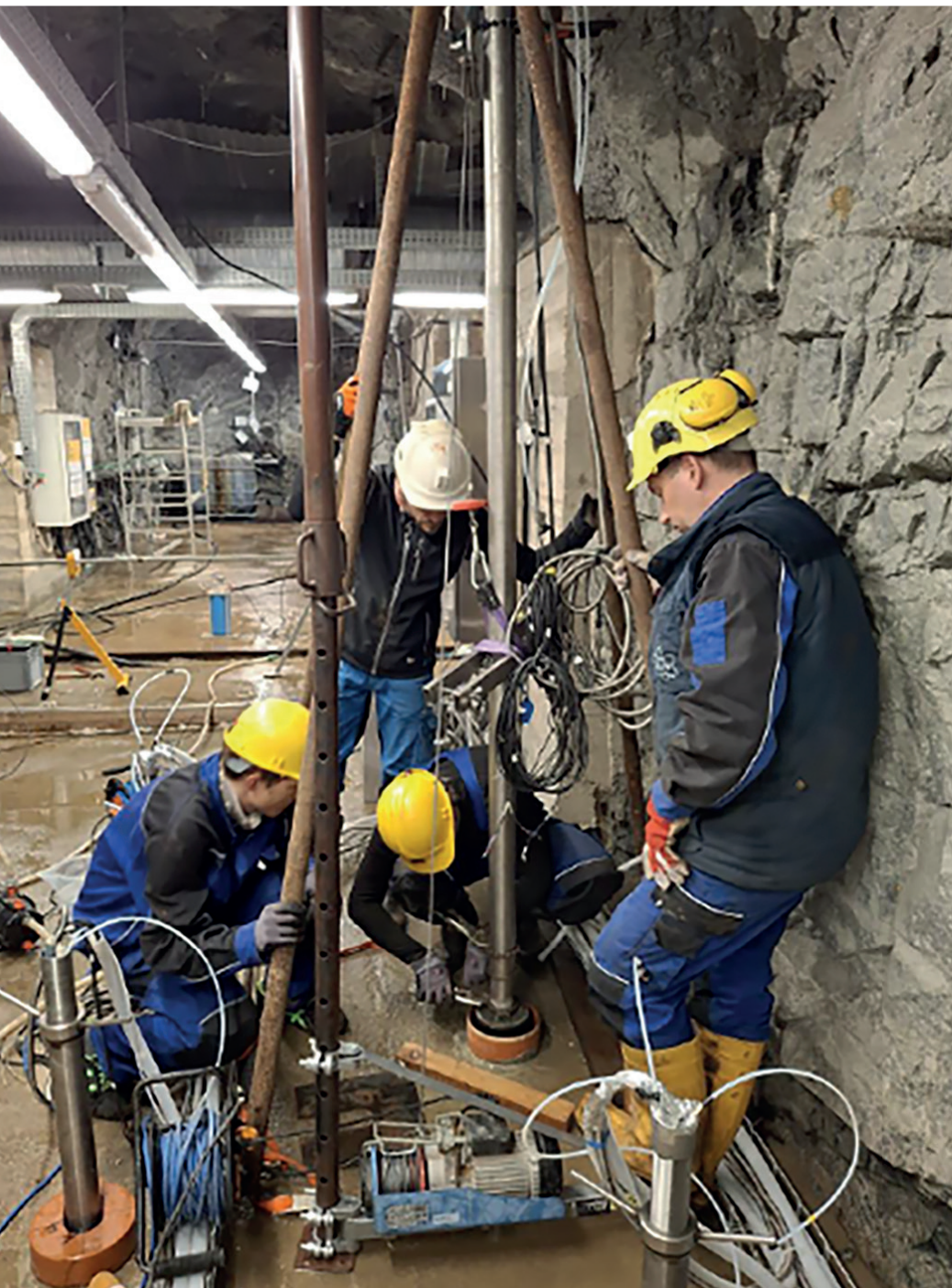
↑ Installation of corrosion modules (2023)
