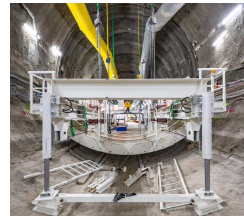
10 m drift lining casting
