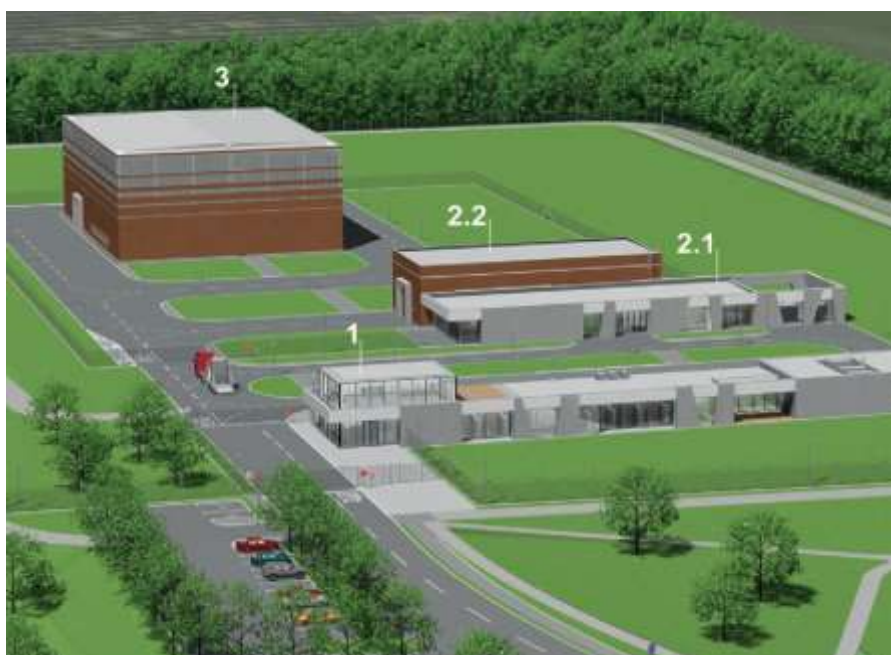
Figure 63 – Above-service facilities: 1. administrative-service facility, 2. technological facilities (2.1 and 2.2), 3. hall above the storage silo [100]
