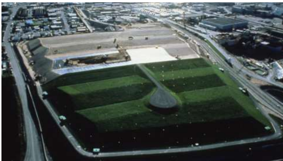
Figure 35 – Cap covering the top of the disposal vaults installed between 1991 and 1997 [79]
