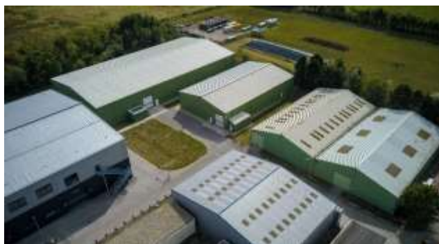
Figure 21 – Interim storage buildings
