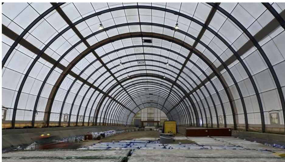
Figure 31 – The disposal facility CIREs [77]
