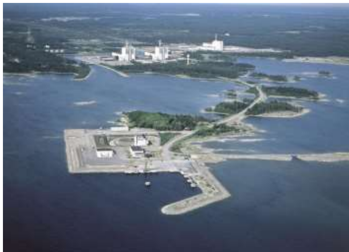
Figure 56 – Forsmark, location of the SFR – Final Disposal facility for Short-lived LILW Radioactive Waste – lies about 50 metres deep in the rock below the sea [97].
