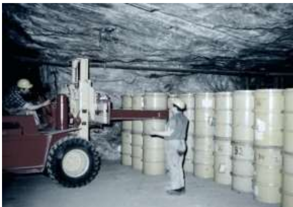
Figure 73 – Vertical emplacement of drums with radioactive waste (LLW) (1967) [117]
