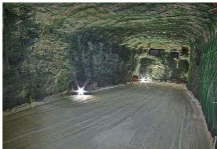
Figure 68 – Emplacement cavity in the east field: Disposal of radioactive waste between 1994 and 1998. (Coverage of waste with salt) [106]
