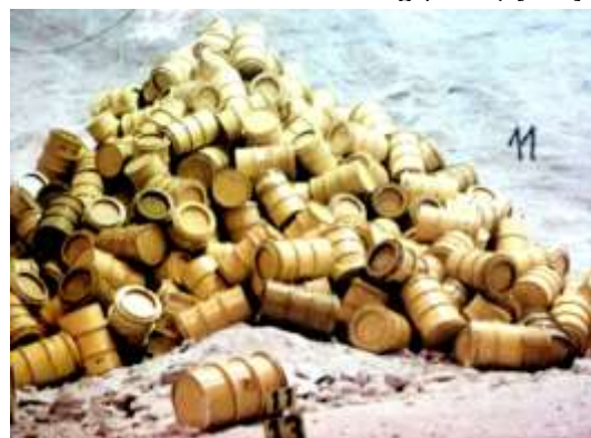
Figure 74 – Drum cone in an emplacement chamber (ILW) [116]
