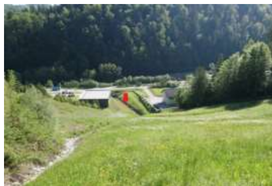
Figure 12 – Lateral drainage channel leads to the main channel of the Jazbec stream (red arrow) [65] [66]
