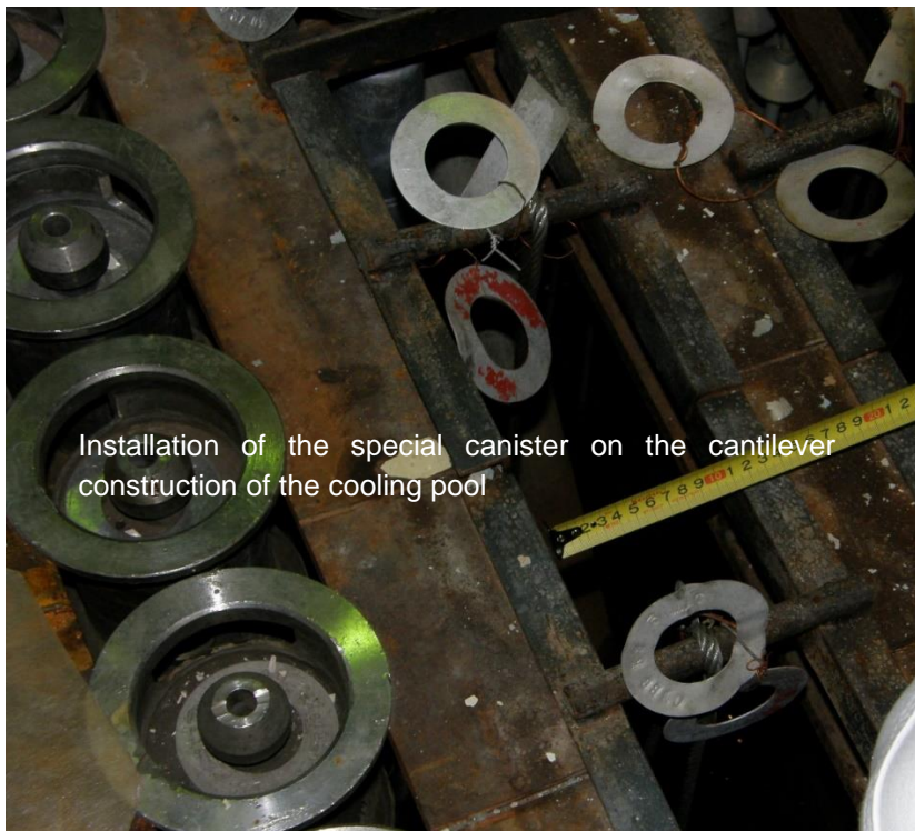
Figure 24: Special canisters for storage of failed spent fuel assemblies in ISF-1 spent fuel pool
