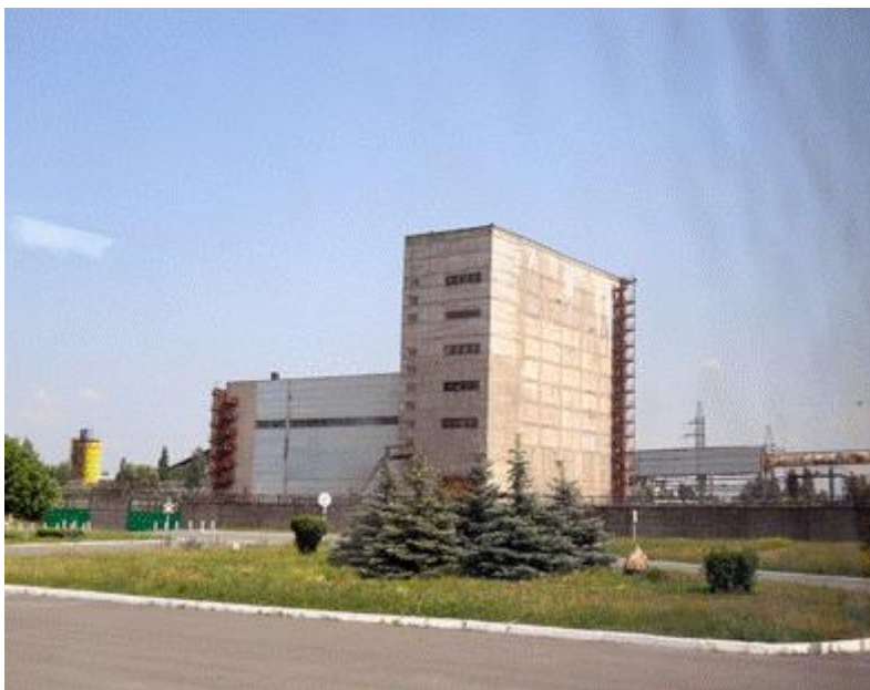
Figure 5 – “Wet” storage facility ISF-1 at ChNPP
