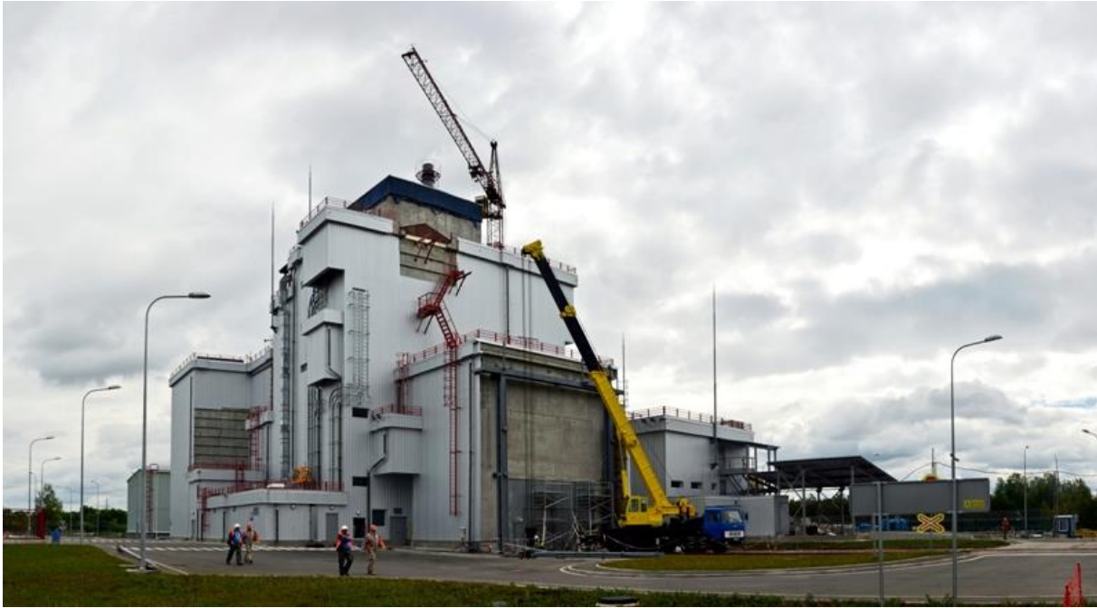
Figure 11 – Spent Fuel Processing Facility (SFPF)
