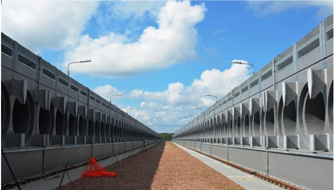
Figure 13 – Area of SNF storage in CSM (SFSA) in ChNPP ISF-2 storage facility
