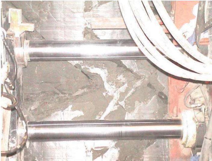
Excavation induced fractures: gallery side-wall
