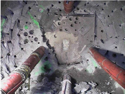
FIRST BENTONITE SLICES ARE REACHED
