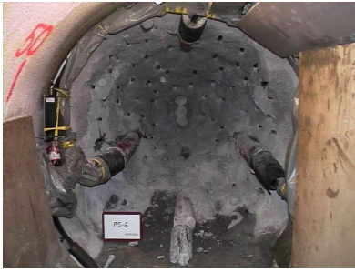
FIRST BENTONITE SLICES ARE REACHED
