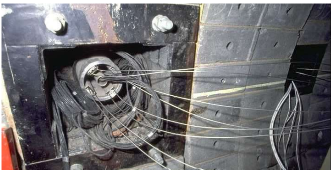
Central borehole with the heating probe
