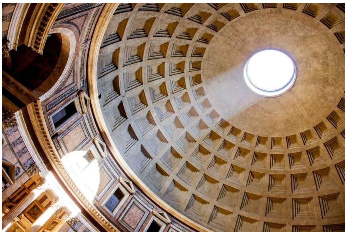
Figure 3-1: Unreinforced concrete dome of the Pantheon in Rome was built in about 120 AD and retains its structural load-bearing integrity 1900 years later. Source: Neil Chapman.
