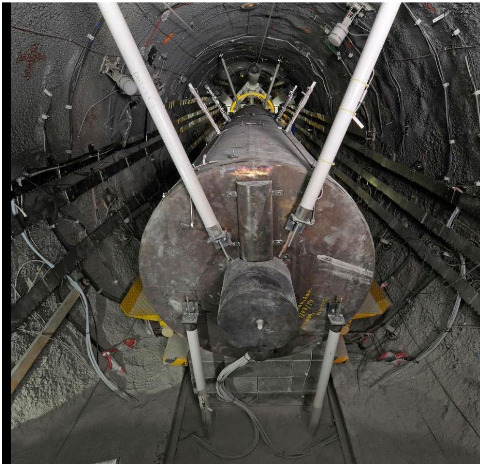
Figure 7-2 Photograph of extensometers used to measure the displacement of heaters in the FE Experiment [10].
