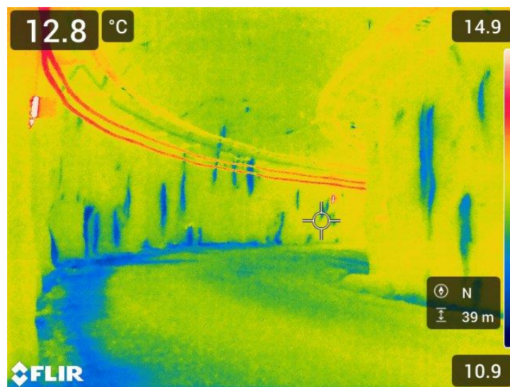
Figure 53: IR-image at around PL3830. Roof and walls are covered with shotcrete. 15.12.2022.
