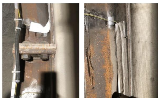
Figure 73: Installation of the sensors for the steel arche section.
