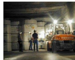
TRU waste package disposal in vaults and test emplacement of borehole disposal in evaporite at WIPP, USA
