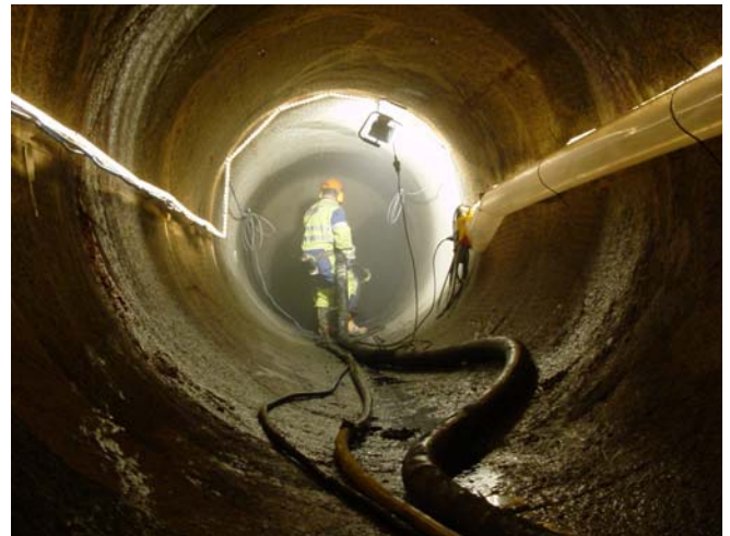
Fig 19 Short Plug Construction at Äspö
