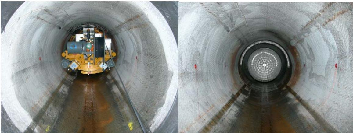
**Figure 11 - The deposition machine has entered the deposition drift (left) - The Super Container is placed approximately 20 meters into the deposition drift (right).**
