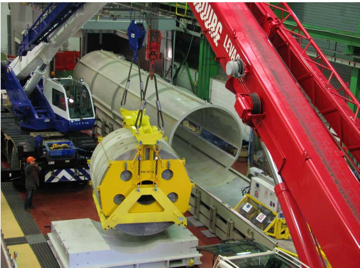
**Figure 15 - Lifting of a set of rings for deposition on the launch table**
