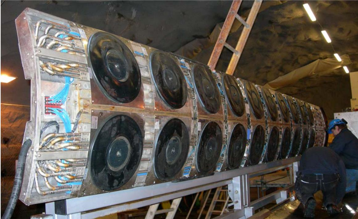
*Figure 9 - Installation of new water cushions on the lifting pallet.*
