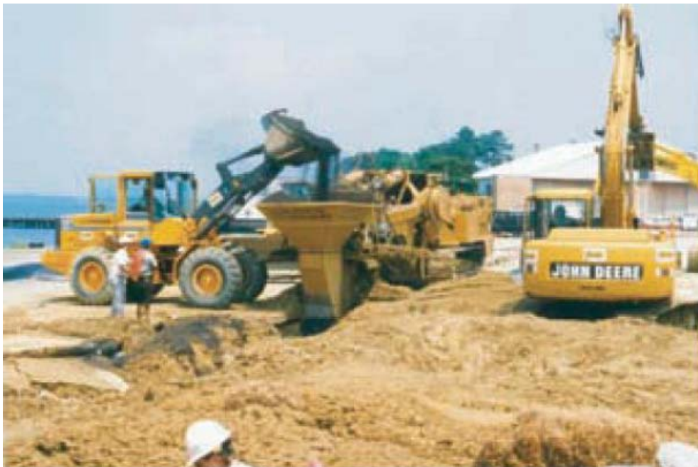
Figure 4.8 (b) Simultaneous excavation and replacement of aquifer material with granular iron as the horizontal trencher advances [43]
