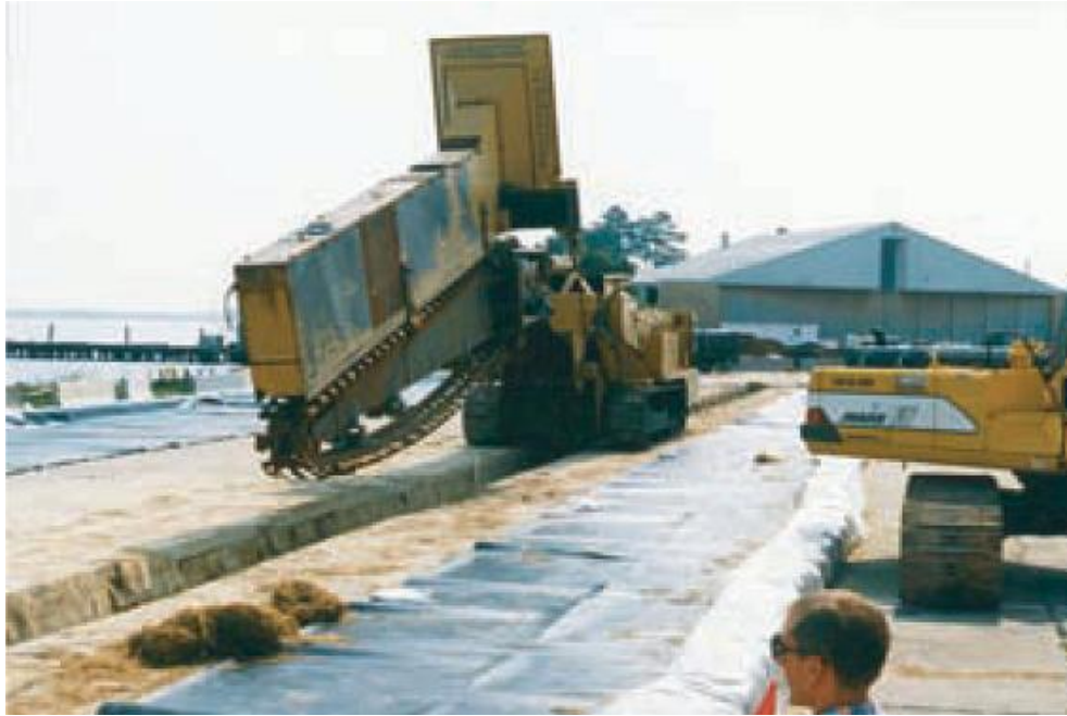
Figure 4.8 (a) Continuous trenching machine used to install a 46 m long, 7.3 m deep and 0.6 m wide granular iron permeable reactive barrier [43]
