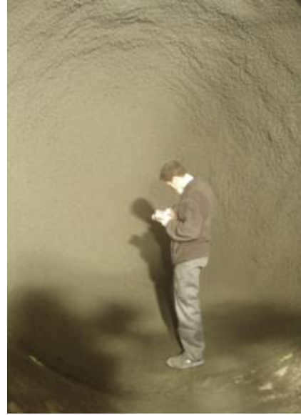
Figure 21: Curved layers of plug
