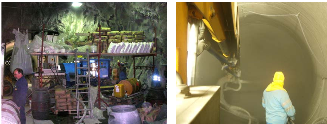
Figure 20: Shotcreting of long plug at Grimsel
