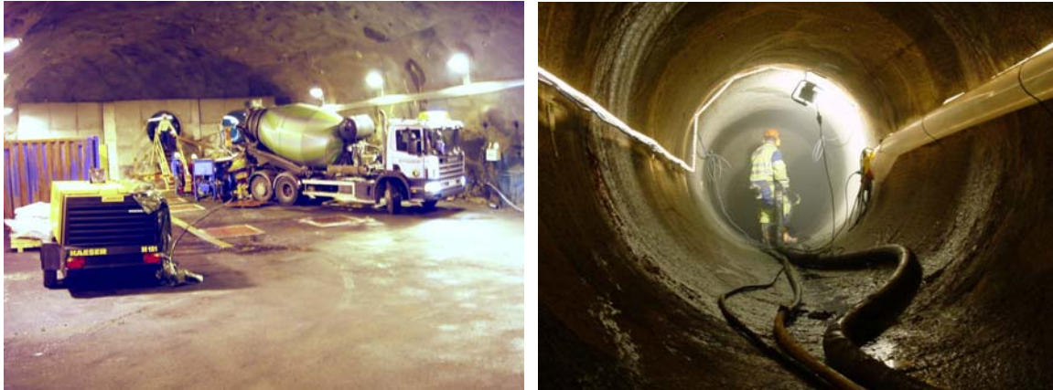
Figure 16: Short plug construction at Äspö HRL
