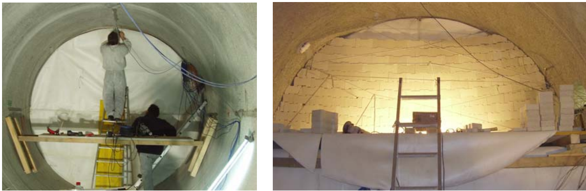
Figure 18: Bentonite buffer construction
