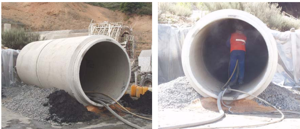
Figure 9: Shotcreting in concrete tube
