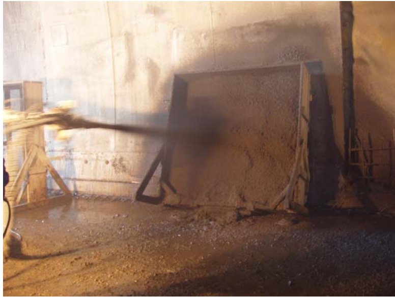
Figure 6: Spraying with robot on panel
