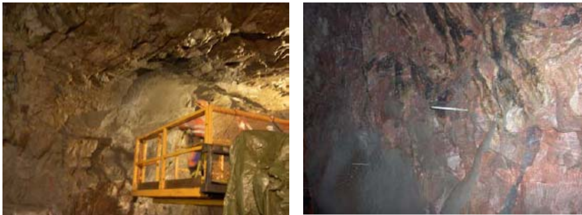
Figure 32: Photo of the equipment for shotcreting at Äspö HRL at level 200 and a close photo of the surface.
