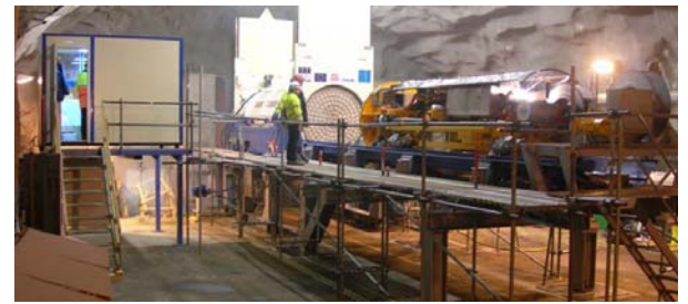
Figure 14: Installation of the KBS-3H deposition equipment at Äspö HRL, Sweden
