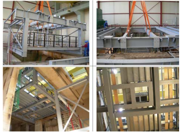
Figure 11: Construction work at test site
