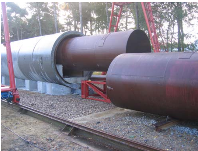
Figure 2: Assembly of the full-scale mock-up
