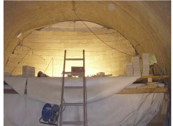
Figure 17: Long plug test. Bentonite buffer construction
