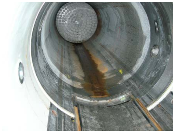
Figure 7: SKB - View of KBS-3H emplaced in the Äspö test drift during the SAT in Feb. 2007
