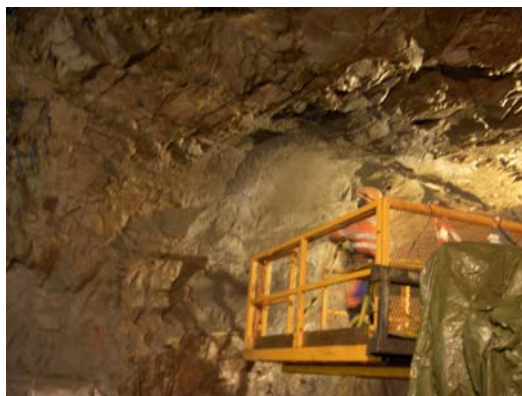
Figure 11: Site test at Äspö URL (Sweden) with low-pH shotcrete for rock support
