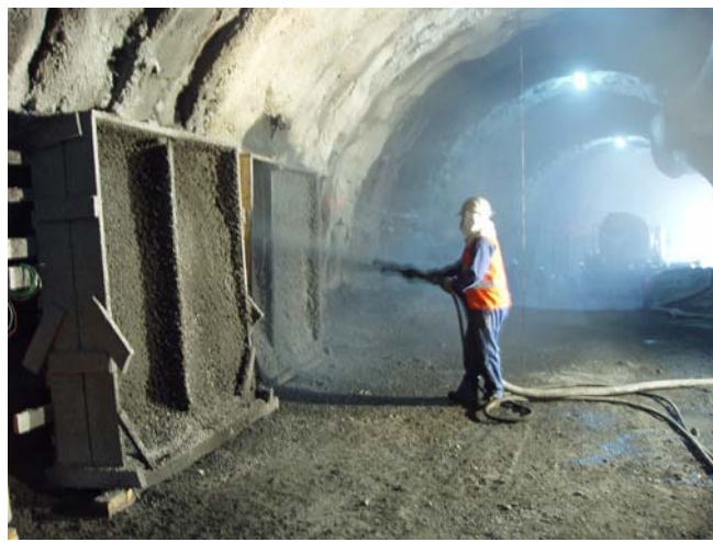
Figure 4: Underground shotcrete test panels at Leon July 2005
