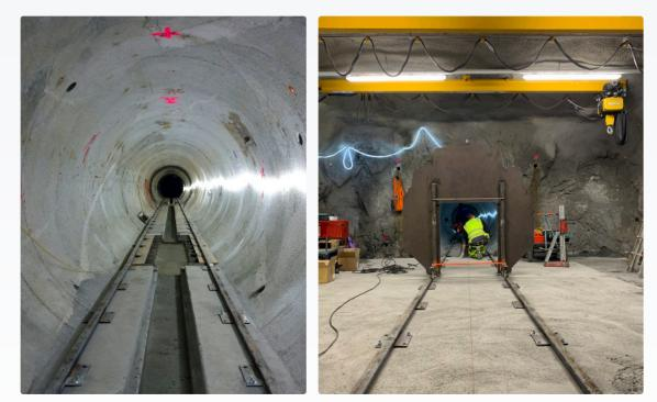
Fig 2: Rail tracks for the auger machine in the emplacement gallery (left) and the niche (right)
