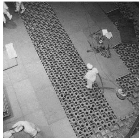
Figure 3: The Latina Reactor Core under construction
