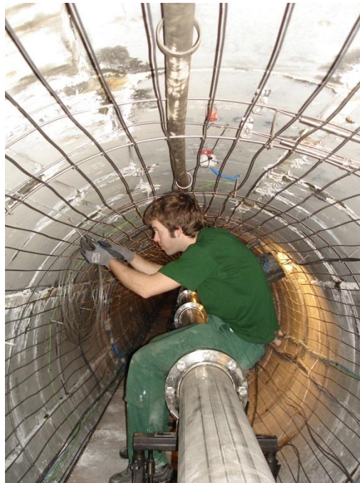
Figure 5-3-2 Installation of fibre optic sensor (single mode for distributed monitoring) inside the PRACLAY Gallery
