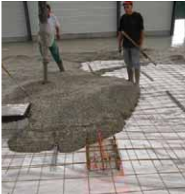
Figure 80: Picture of concrete slab pouring when concrete embeds reference sensors
