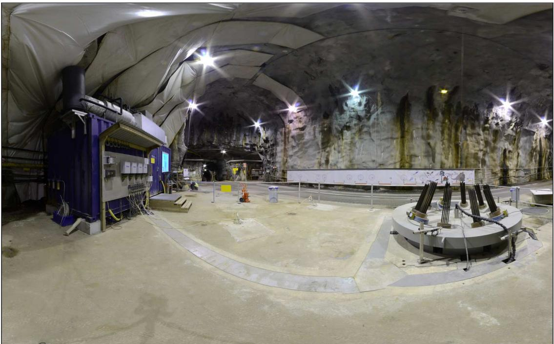
Figure 3.1: TBM assembly hall interior. Gas laboratory (left) and Lasgit's retaining lid with anchor cables (right) (Cuss et al. 2010).
