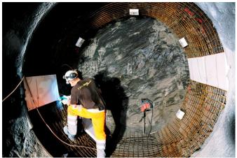
Tunnel support made with steel nets and shotcrete
