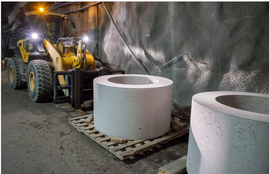
Fig. 28 Carrying of ring blocks in Onkalo by the wheel loader.
