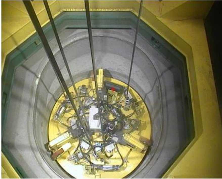
Fig. 32. Installing the top solid blocks, seen by BIM dome camera.
