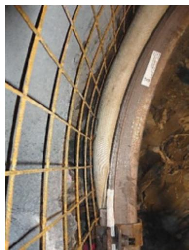
Fig. 16b: TH 25 arch, Bullflex, wire mesh K 196 before shotcrete 5 cm
