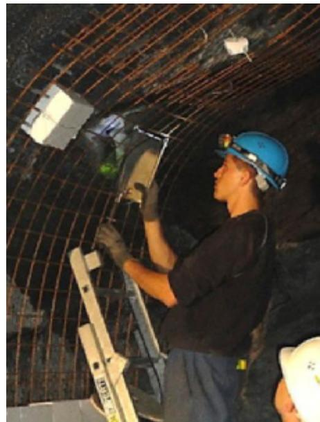
Fig. 49a: Installation of a strain gauge
