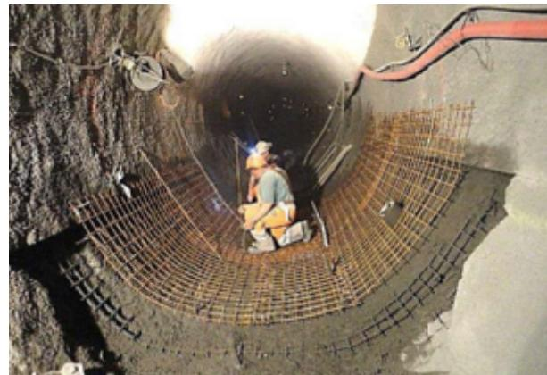
Fig. 37: Installation of the 2nd wire mesh
