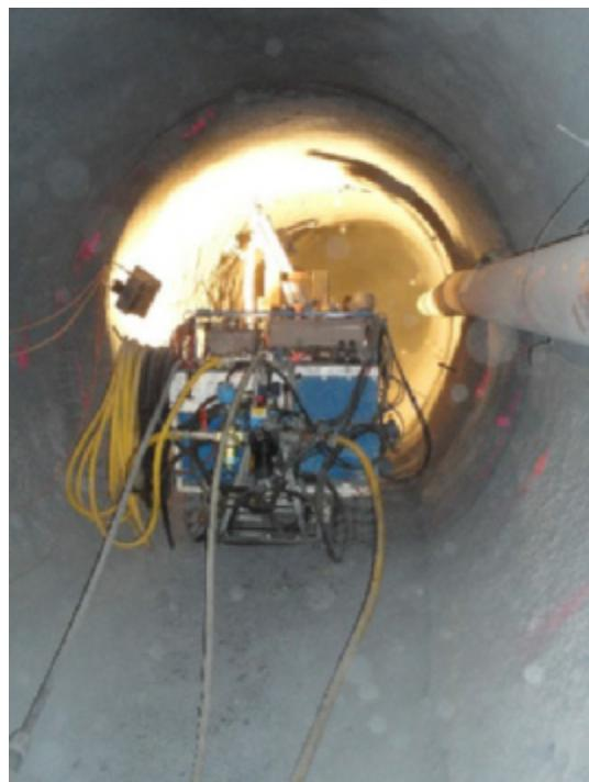
Fig. 40b: Grouting of additional rock bolts
