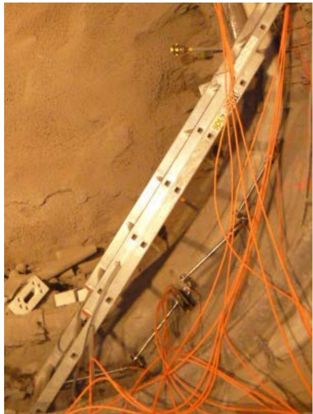
Fig. 50a: GM 43.20 installation of crackmeter
