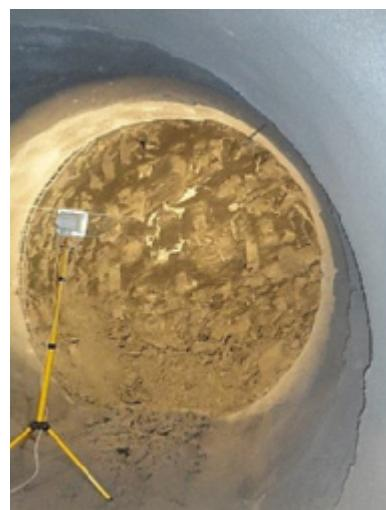
Fig. 17b: Profile excavation and support after excavation and roadheader profiling
