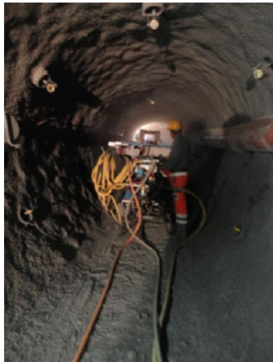
Fig. 40a: Boring of additional rock bolts
