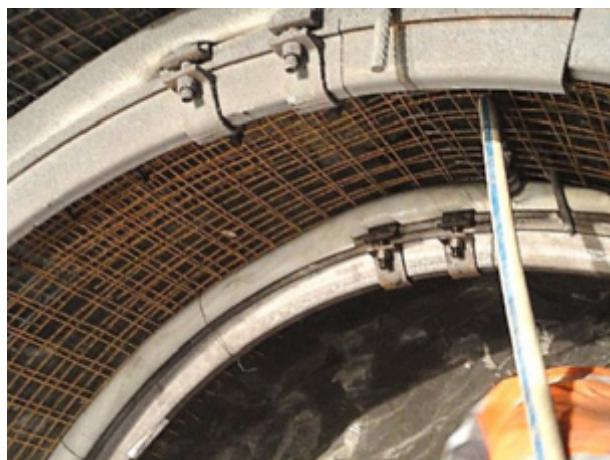
Fig. 22: Bullflex grouting
