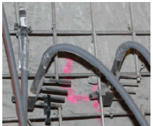
*Fig. 6: Corrosion monitoring system*
