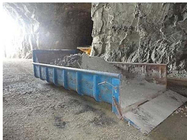
Fig. 11: Deconstructed concrete, removed to inert waste controlled landfill
