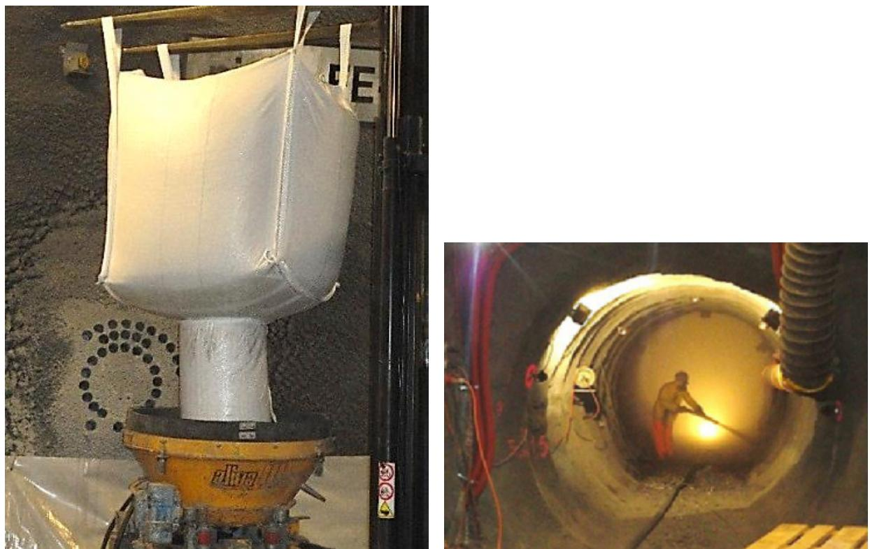
Fig. 27: Shotcrete conditioning, handling and installation
