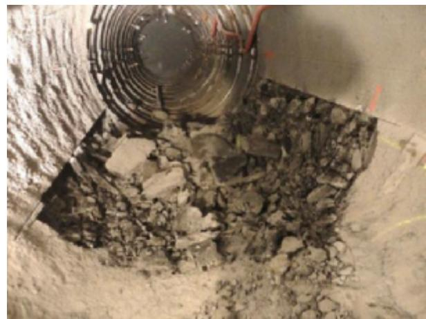
Fig. 32: Deconstruction of shotcrete
