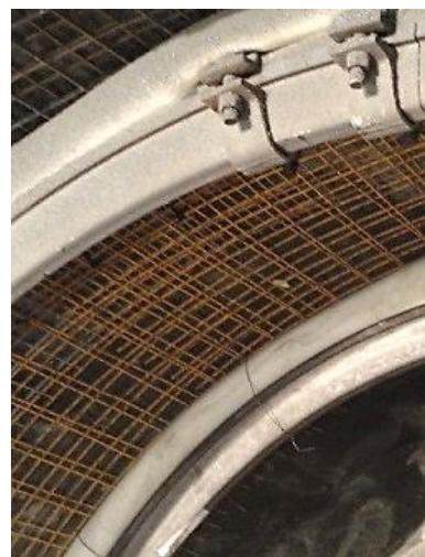
Fig. 18b: TH 25 arch, Bullflex, double wire mesh lining K 196
