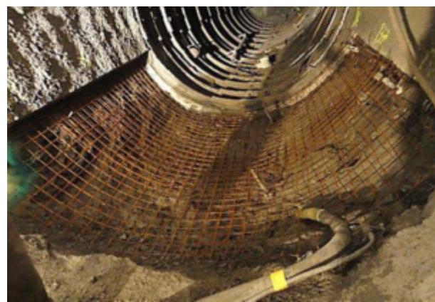
Fig. 36: Installation of the 1st wire mesh
