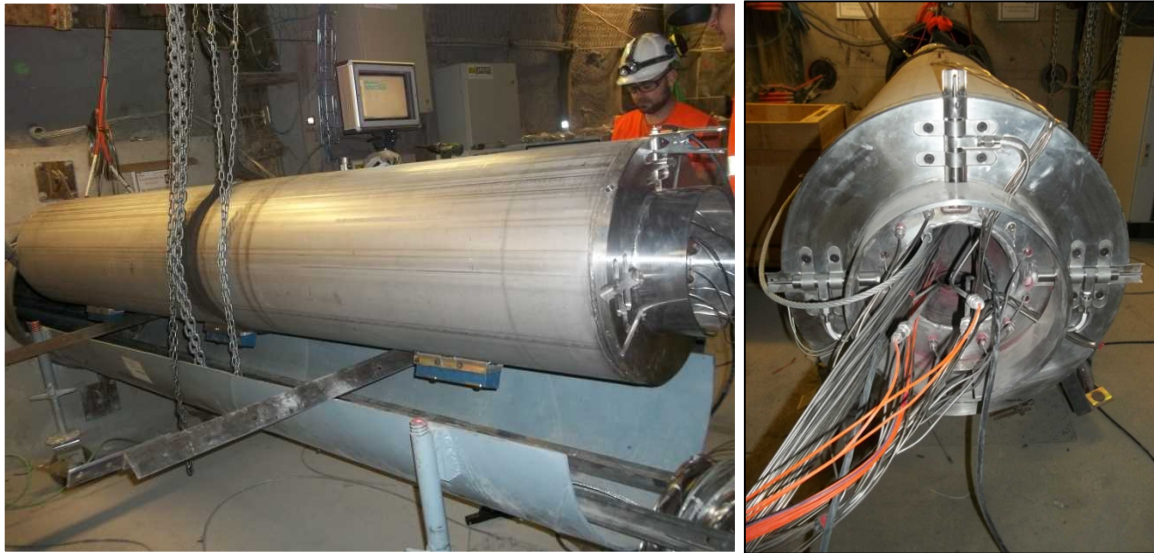
Figure 6: (left) View of a heater element when it is installed. (right) View of a heater/sleeve distance variation sensor section
