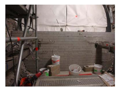
Fig. 2.5 General layout of the NSC experiment in the MHM-URL and seal construction in the drift using bentonite-sand blocks and bentonite pellets /DEL 15/
