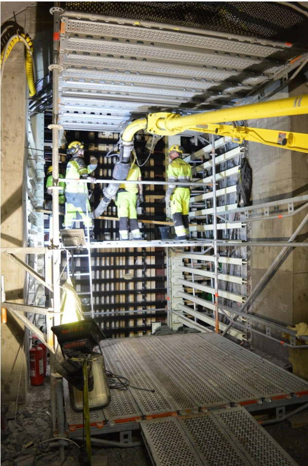
Figure 1. Emplacement of the plug concrete.
