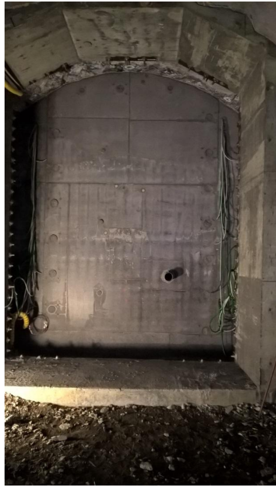
Figure 2. Plug appearance after formwork removal (prior to contact grouting and pressurization).
