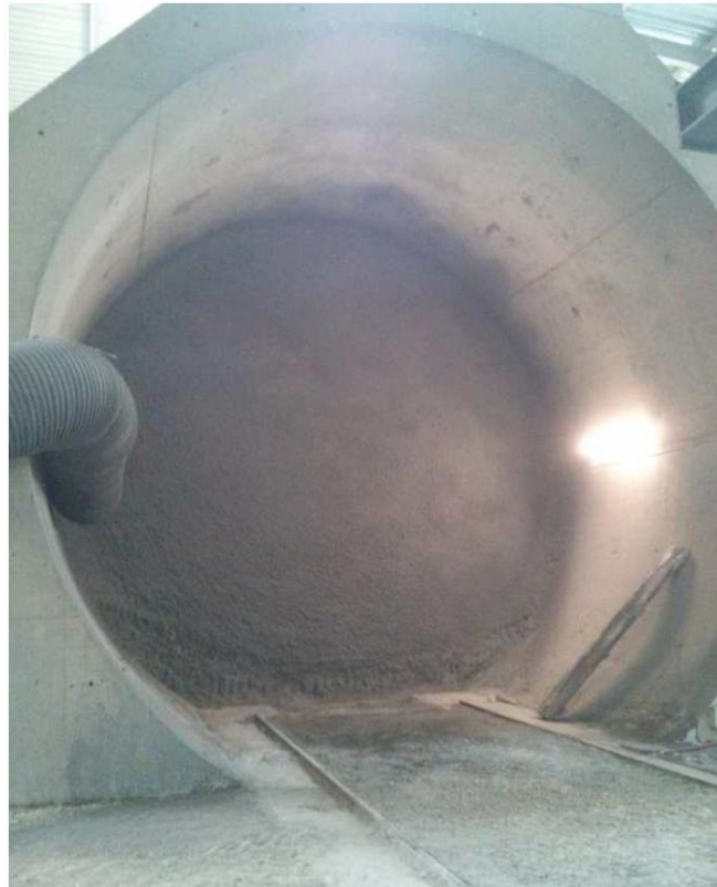
Figure 5.3: The low pH Shotcrete wall completed
