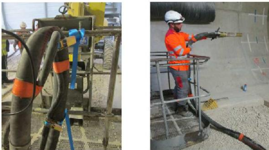
Figure 4.2: Fixing of spraying gun on platform
