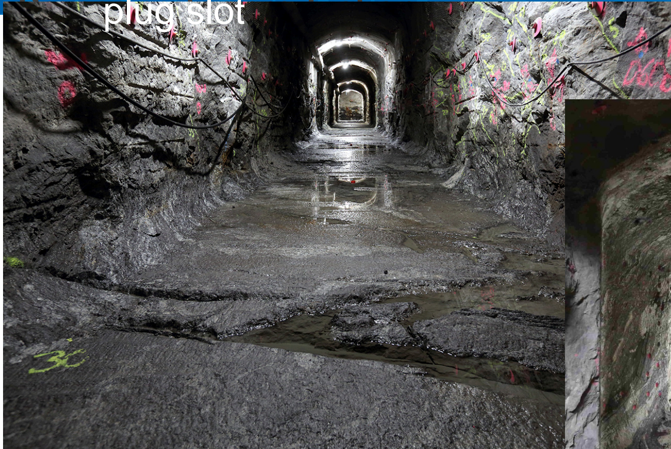
Demonstration disposal tunnel
