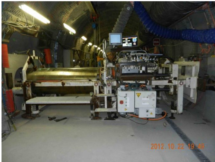
Drilling of a 25 m long cell.
