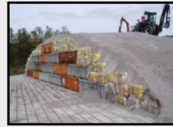
First type: landfill repository for VLLW, Sweden (In Ukraine Buriakovka)
