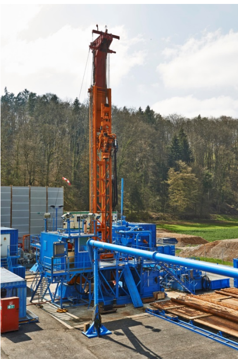
Site investigation drill rig.
