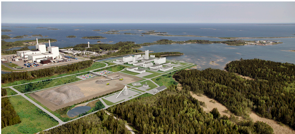
Aerial photo and montage of the planned site of the Spent Fuel Repository (centre) at Forsmark.
