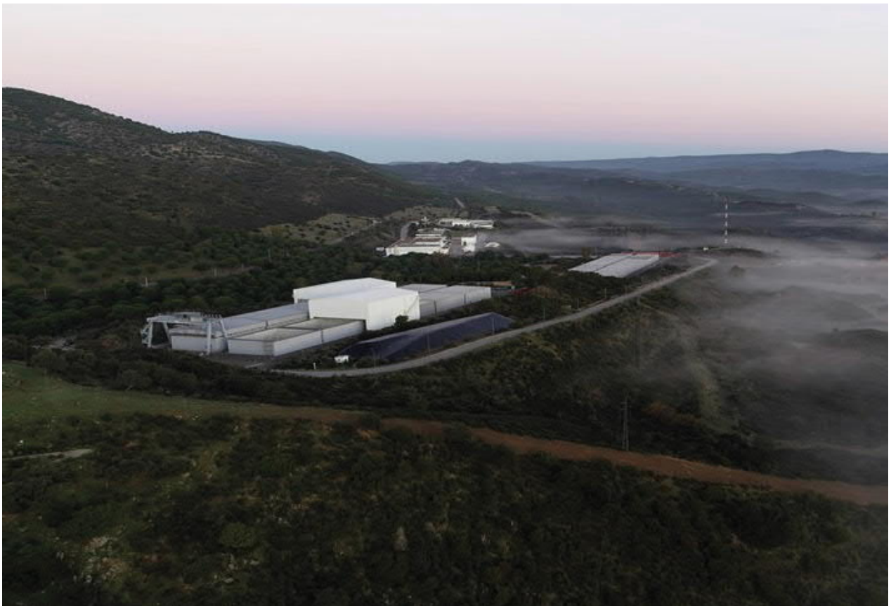
Aerial view of El Cabril repository for LILW and VLLW (Enresa)
