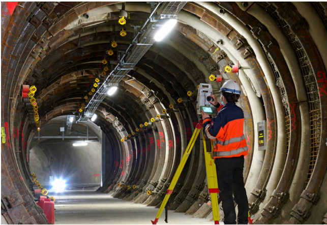
Interior view of the Mont Terri rock laboratory ( mont-terri.ch )
