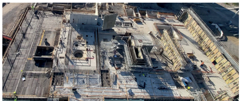
Construction of the encapsulation plant at ONKALO® site, photo Posiva Oy
