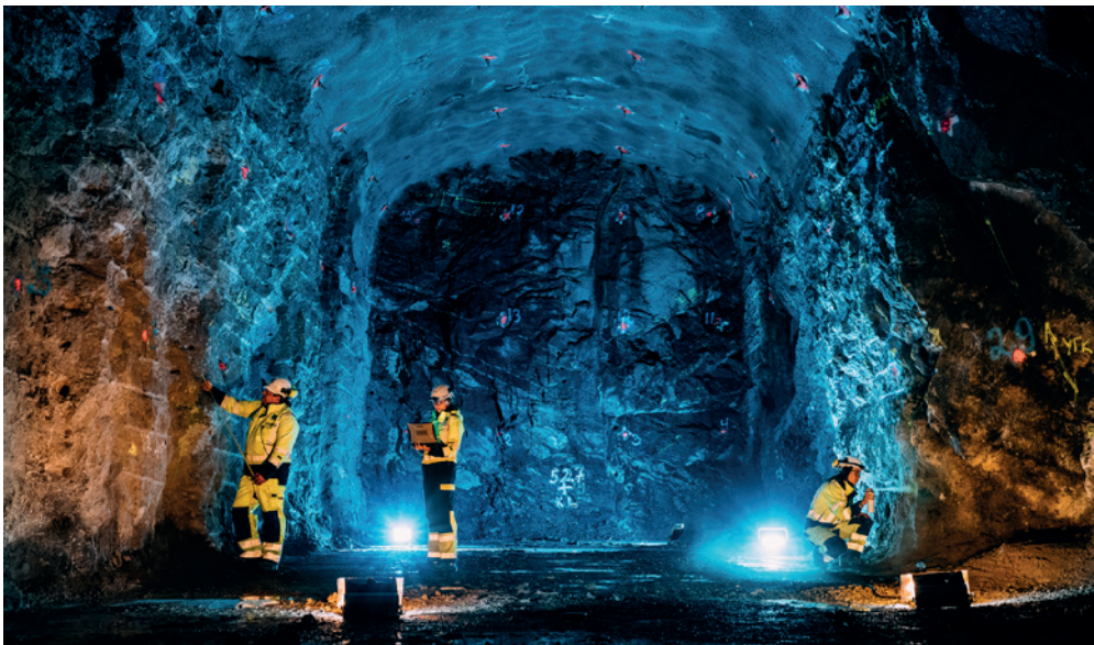
Construction in Posiva’s final disposal facility is ongoing, photo Posiva Oy
