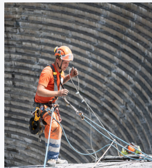
Worker preparing the blasting for the basement excavation 2019 (© KWO)
