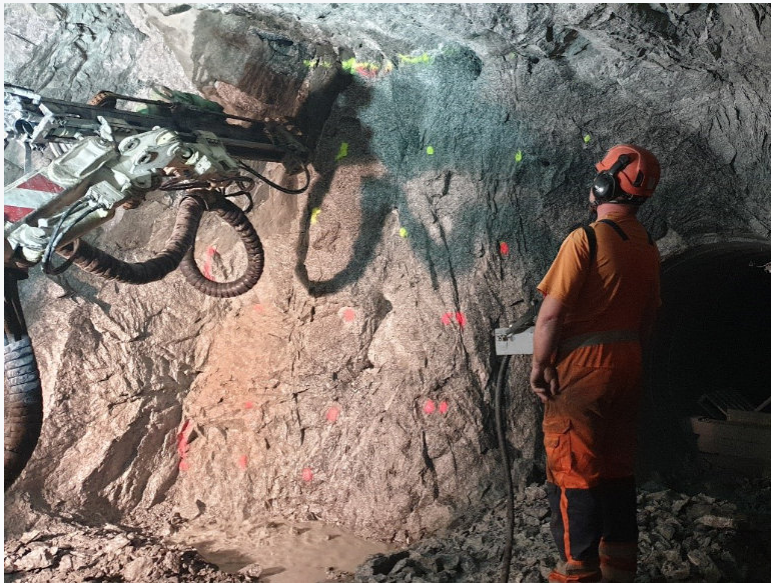
Drilling blasting holes (left)
