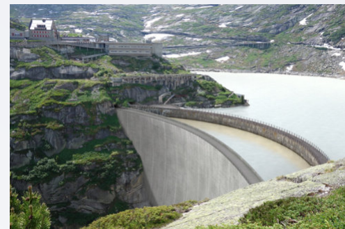
Visualisation of new dam in front of the old structure (© David Ormerod, KWO)
